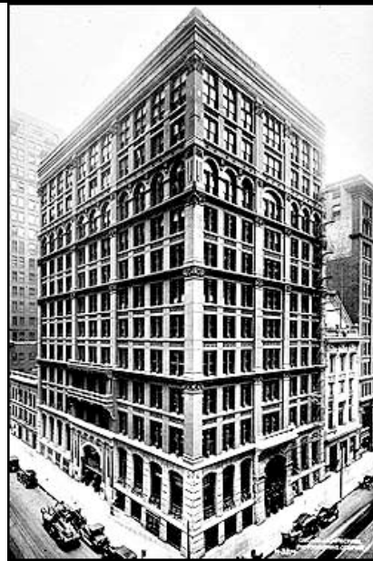
Name - Home Insurance Building Location - Chicago, Illinois Height - 138 feet Floors - 10 Cost - undetermined Materials - steel
