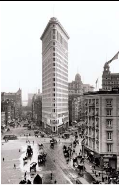
Name - Flatiron (or Fuller) Building Location - New York, New York Height - 285 feet Floors - 22 Cost - $41 million then, $800 million in 2005 Materials - steel and stone
