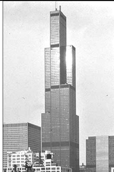
Name - Sears Tower Location - Chicago, Illinois Height - 1454 feet Floors - 110 Cost - $150 million then, $600 million in 2005 Materials - steel and aluminum
