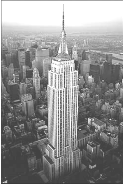
Name - Empire State Building Location - New York, New York Height - 1250 feet Floors - 102 Cost - $41 million then, $500 million in 2005 Materials - steel, stone, bricks and aluminum
