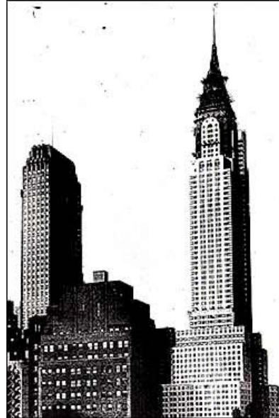
Name - Chrysler Building Location - New York, New York Height - 1046 feet Floors - 77 Cost - $20 million then, $250 million in 2005 Materials - steel and bricks
